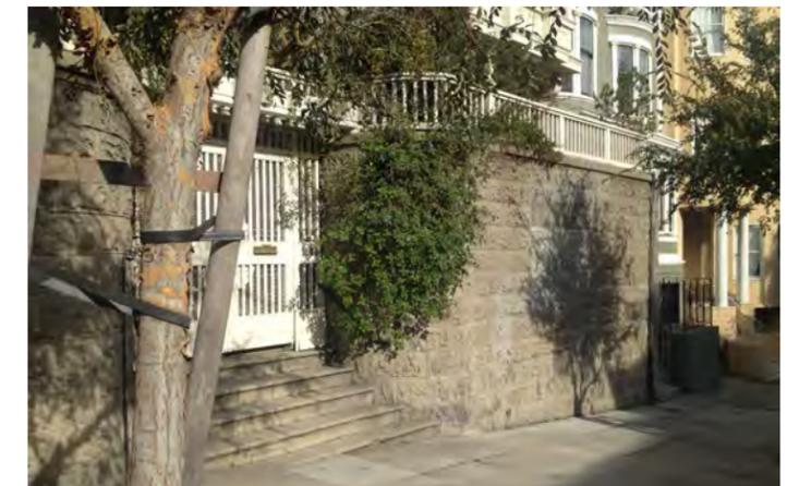
A structural, reinforced concrete retaining wall is covered by a sculptured veneer treatment and further softened with a railing and foliage.
