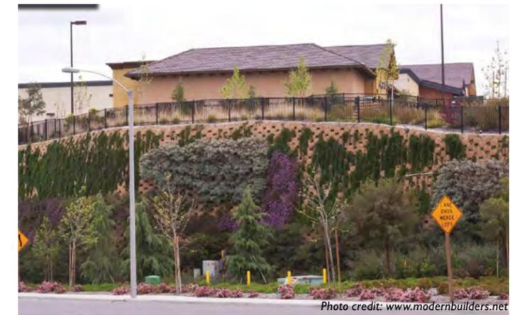
The VERDURA Living Retaining Wall system is a fully plantable block wall that is Caltrans approved.
